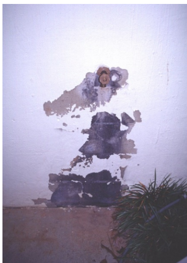
Figure 5. Repair plumbing leaks as quickly as possible. Moisture attracts termites to the structure.
