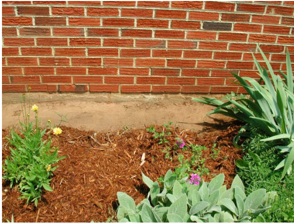
Figure 4. Leave a 12-18-inch bare zone (i.e., pull back the mulch next to the foundation to prevent providing a bridge to subterranean termites over the termiticide-treated zone).
